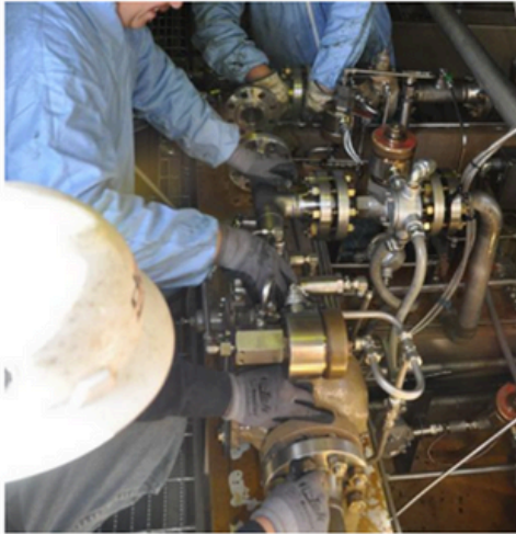
Installing the new electronic fuel valve
