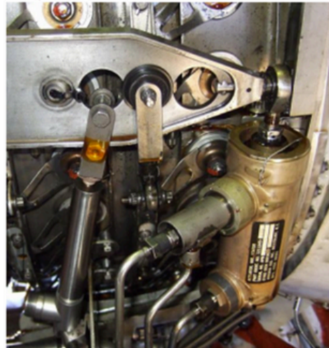
New VSV feedback LVDT installed
